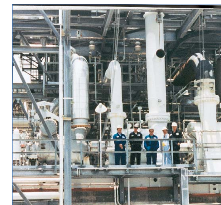
Surplus equipment rerated and installed
