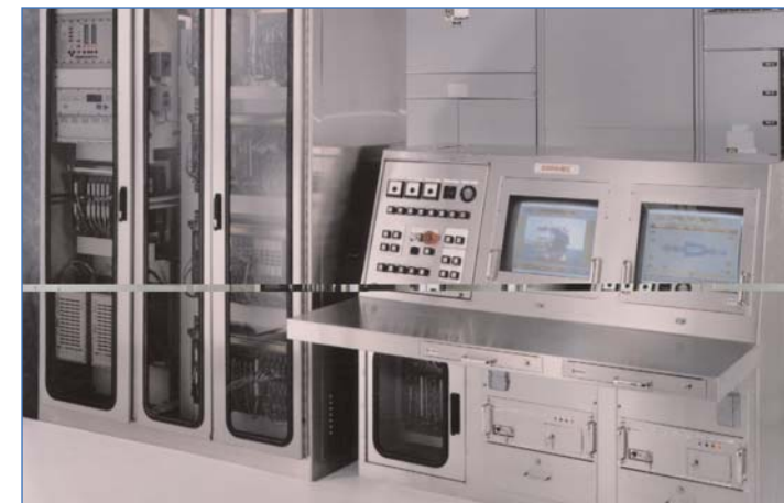
GE's Conmec marine environment gas turbine control system
