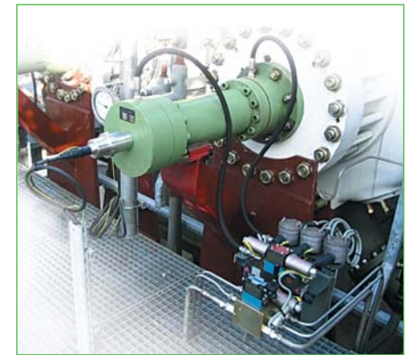
Figure 3: Hydraulic actuator
